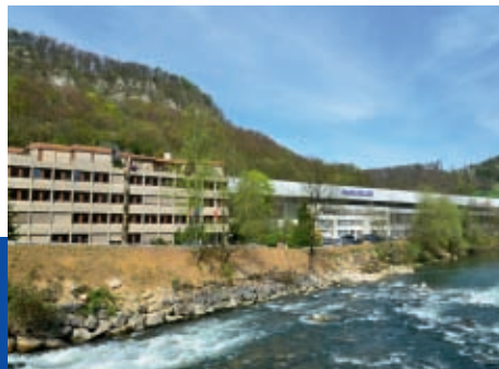
HAEUSLER headquarters in Duggingen, Switzerland
